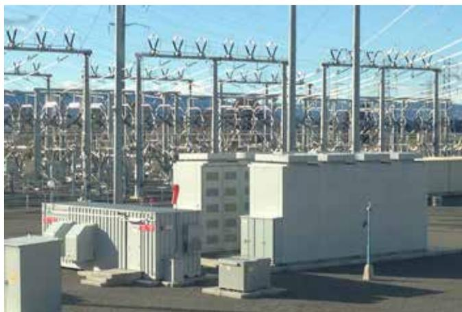
*The sodium sulfur battery located at the Pacific Gas and Electric facility in Vaca-Dixon, CA was the first to provide services to the ISO market. Utility scale energy storage such as this one offers significant flexibility in balancing the grid under a variety of conditions. The potential operational benefits include:*
