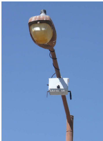
Figure 5 Power SG Data Concentrator Attached to a Street Lamp
