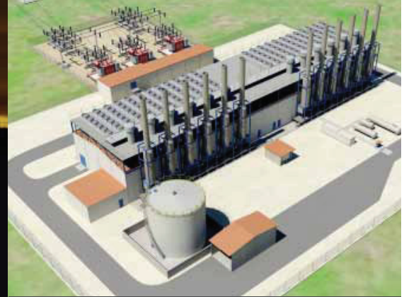
Wärtsilä Flexible Grid Stability Plant, 100 MW, optimized for peaking and reserve power applications running on liquid fuel oils and/or natural gas.
