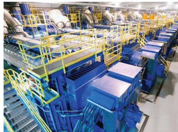
■ Fig.2 – Power plants based on Wärtsilä gas engines have been optimized for maximum flexibility.
