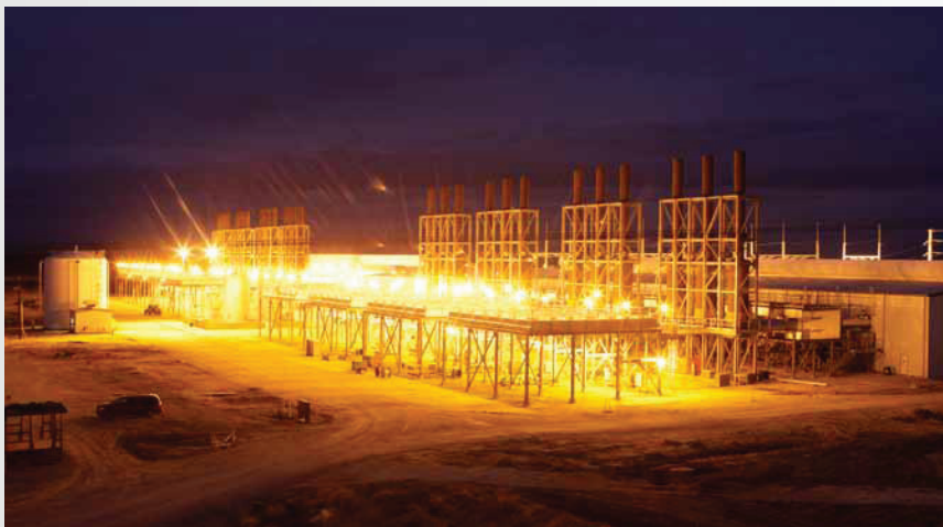
■ The 202 MW STEC power plant in Nursery, Texas.
