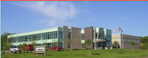
Headquarters, Operations, and Factories - Warrendale, PA
