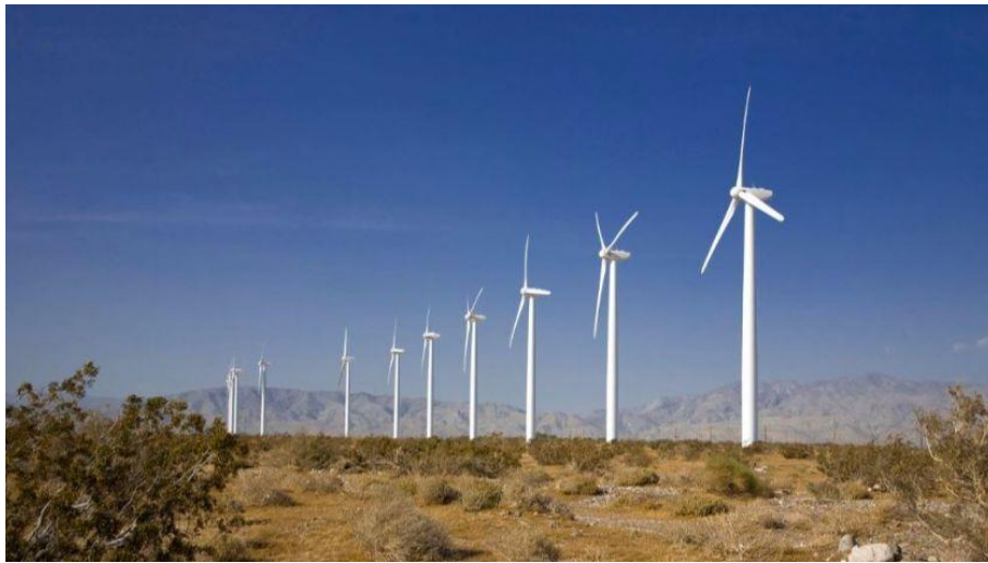
Figure 7. Tule 131.1-MW wind farm (Source: Avangrid Renewables)
